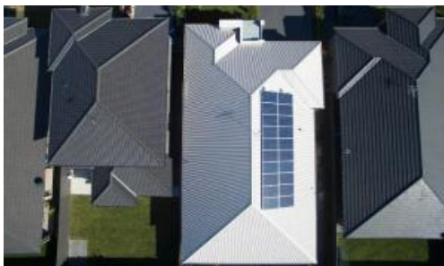
In general, lighter coloured roofs are cooler
